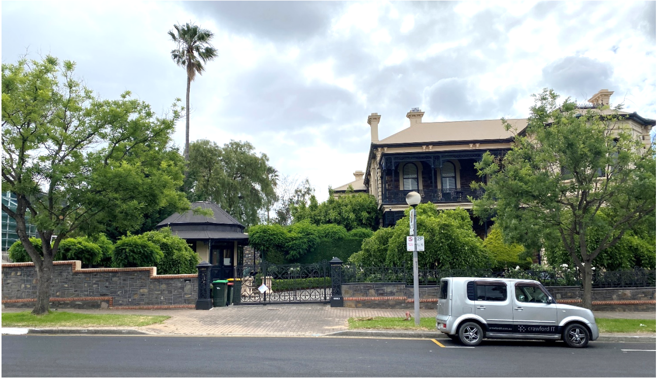
Figure 3.1 - subject site viewed from East Terrace
